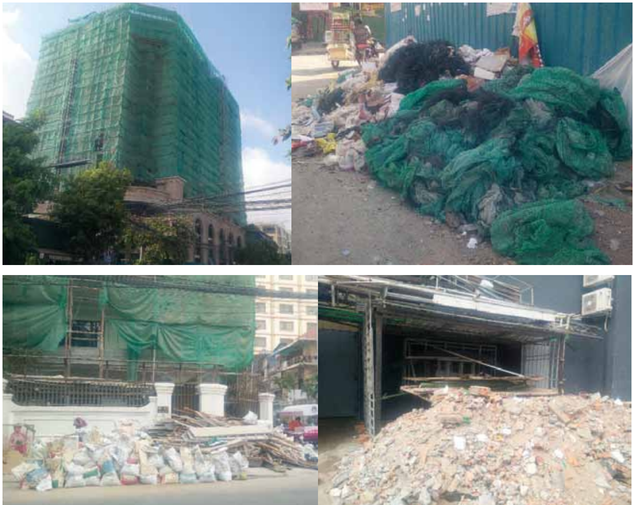
Figure 17 Generation of C&D waste (Source: COMPED)
